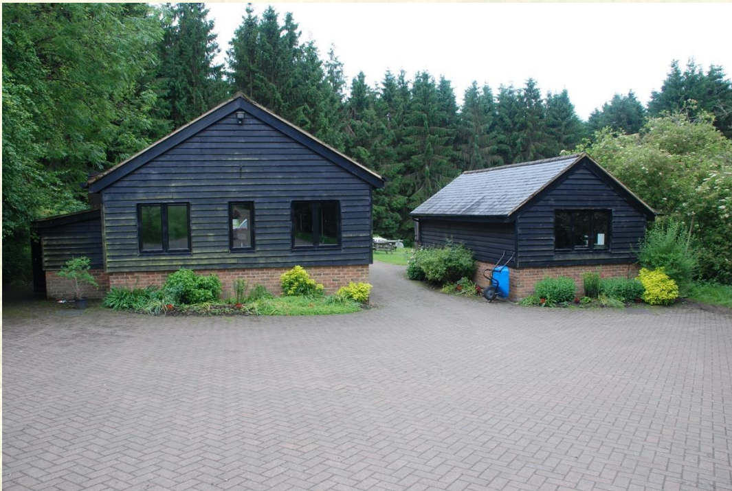
The barn and café building
